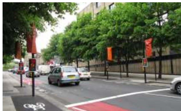
The staggered Toucan across the gyratory at George Street adjacent to the police station. Hoods have now been removed and the lights are synchronised with Dalton Square signals.
