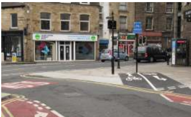
The Stonewell crossing is soon to be widened and Toucanised so cyclists will no longer need to dismount to cross the gyratory.
