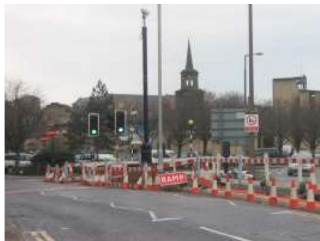
Working on the crossing
