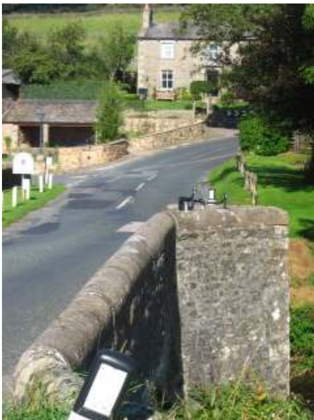
Condor Mill Bridge with pedestrian refuge
