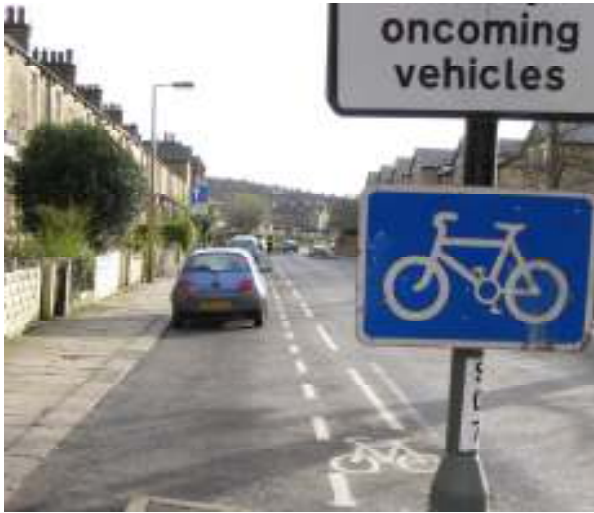
Pinch point and, dangerously positioned cycle lane on Willow Lane
