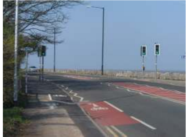
Toucan crossing: cyclists going downhill use the on-road cycle lane; cyclists going uphill use the shared-use pavement
